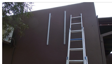
Cut unistruts the same length as condenser height and install
