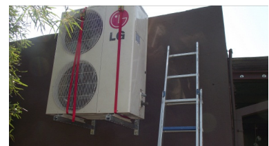
Install cantilevers and lower condenser onto cantilevers
