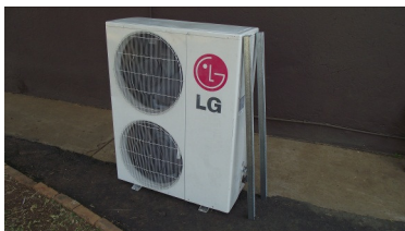
Cut unistruts the same length as condenser height and install
