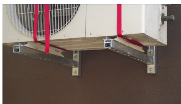
Install cantilevers and lower condenser onto cantilevers
