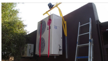
Strap H bracket on condenser
