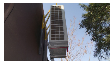
Turn lever clockwise to lift condenser
